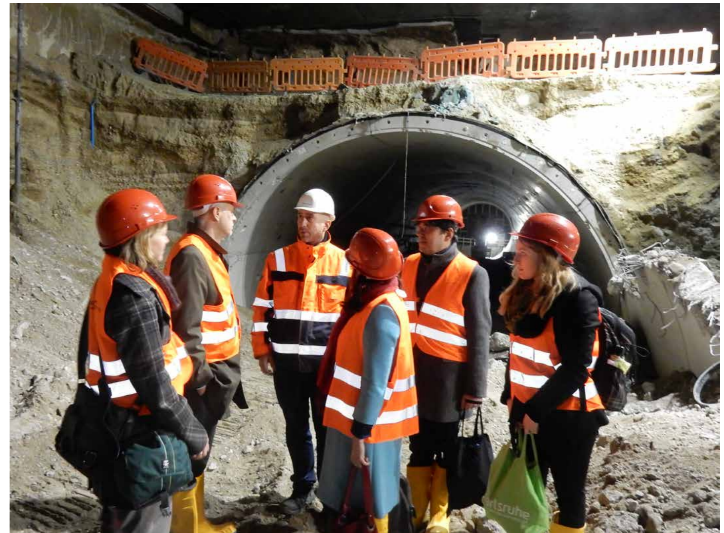
Leader of the Council and Deputy Chief Executive from Nottingham (on the left) on construction site tour under Karlsruhe's market square in 2016. Photo: Liane Wilhelm, City of Karlsruhe
